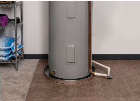
Water Heater Drain Pan w/ CPVC Fitting A drain pan is always recommended for installation in a finished room or attic where you would want your flooring or ceilings protected.
